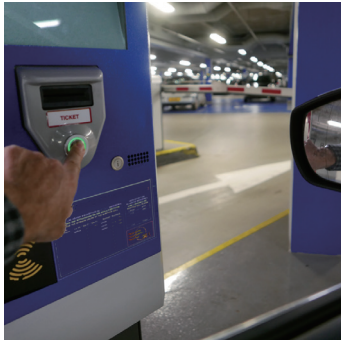
Networking data from parking systems, ticket machines, and so on
